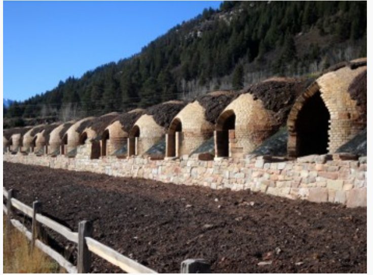
BRS hand cut about 20,000 bricks to fit the ovens' distinct shape.
