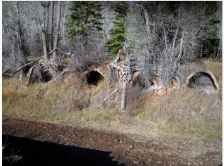
Deterioration and overgrowth had to be cleared before BRS could begin imagining what the original ovens looked like.
